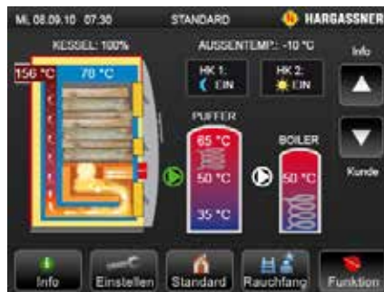
Boiler in Full-Load: Display shows a working boiler. HWT and Accumulator are being loaded already. Heating Circuits ensure required temperature in each living-area.
